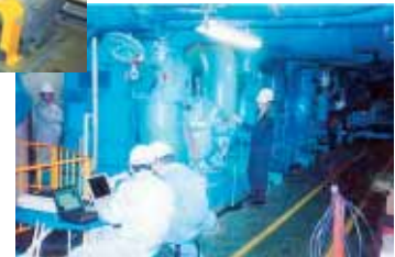
Conducting a pump efficiency measurement at an actual plant by applying a technique developed by CJ*
