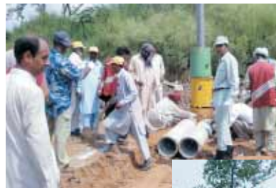
Construction of drainage pipes and vents at the landfill site in Islamabad
