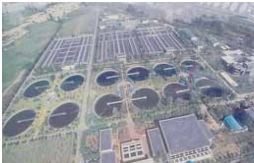
Bird's-eye view of the No. Seven and No. Eight sewage treatment plants
