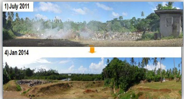
Rehabilitation of Kalaka Dumpsite (Tonga)
