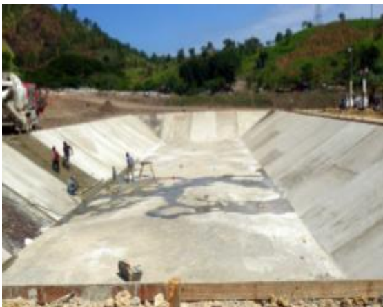
Photo 2. Leachate pond construction & Environmental Management (Surface Water monitoring & Leachate control)
