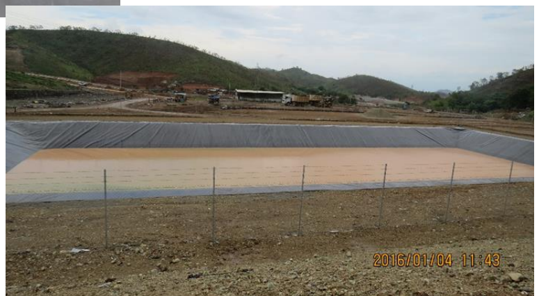
Completed and fenced leachate pond
