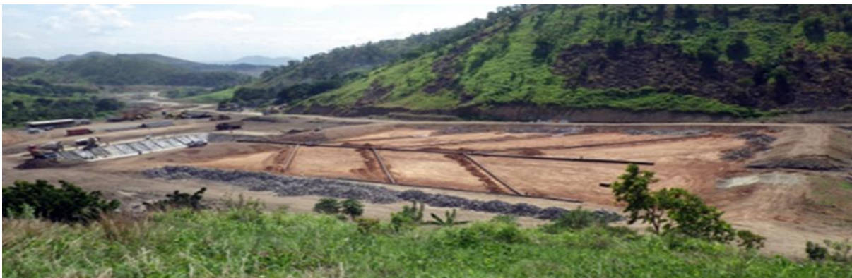
Photo 1. The Completed cell ready for operations
