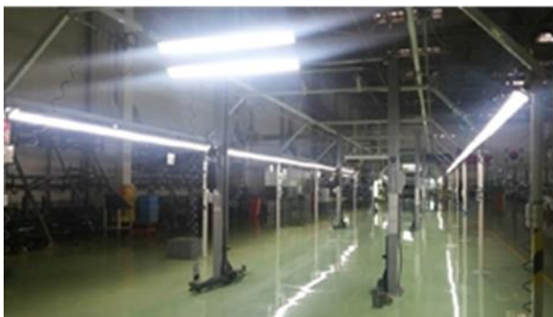
112Vt fluorescent lights were replaced with 72Vt LED (70pcs)
