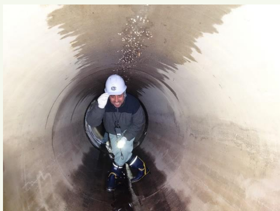
Practice of sewer pipe inspection
