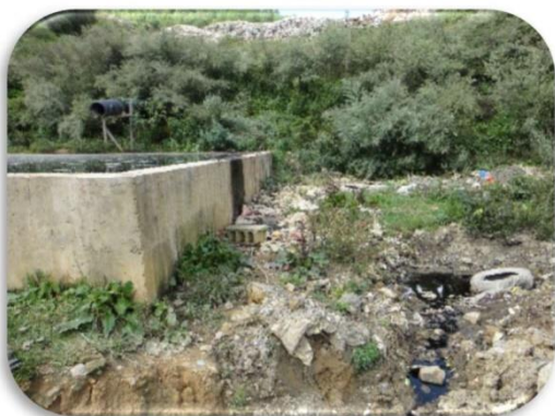
Photograph 1-3: Leachate cannot be treated by a reservoir alone, and causes water pollution
