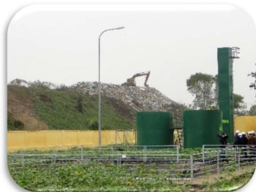
Photograph 1-4: Leachate treatment facility at a landfill disposal site
