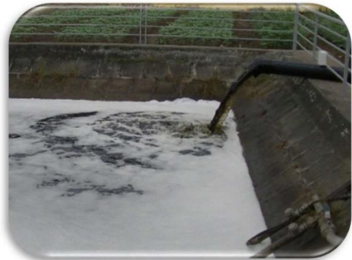
Photograph 1-2: Leachate from landfill disposal sites is dark-colored because the wastes contain raw garbage
